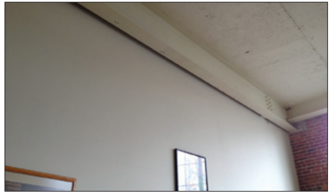
Figure 3. Beam parallel to wall partition.
