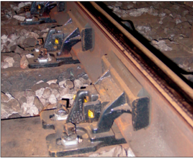
Figure 4. Resilient track fastener.
