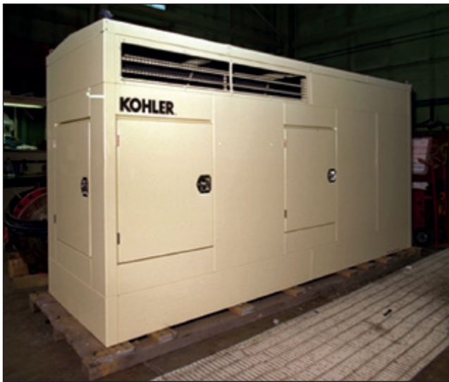
Figure 7. Example of a manufacturer-supplied noise control enclosure on a diesel generator.
