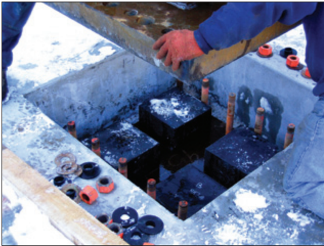
Figure 5. Base isolation pad.
