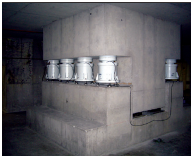
Figure 10. Case Study 3: Air-spring-supported inertia block.
