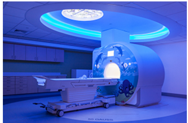
Noise transmission from above-grade MRIs was a concern in designing patient rooms at Boston Children's Hospital. Photo Credit: Emily O'Brien Photography
